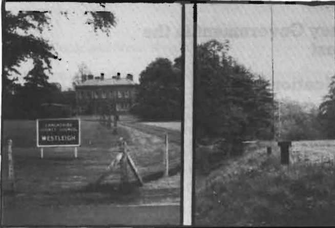
Westleigh, showing aerial and ventilation pipe emerging from the bunker at the back.
