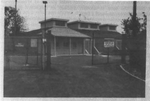
Top Centre: The massive UKWMO/ROC bunker, Langley Lane, Goosnargh, with refurbishment (pipe lagging) going on one Sunday in May, 1982.
