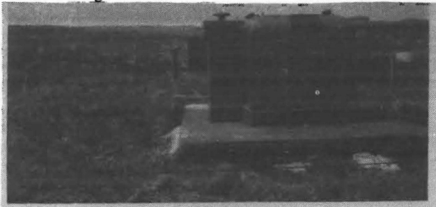
Royal Observer Corps monitoring post, Kendal. (See appendix B).
