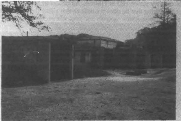
Mystery bunker, Whittingham Lane, Goosnargh. Possible entrance to the extensive tunnel network reported to centre on the massive UKWMO bunker at Langley Lane, several hundred yards away.
