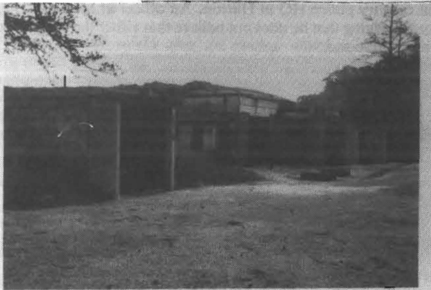
Mystery bunker, Whittingham Lane, Goosnargh. Possible entrance to the extensive tunnel network reported to centre on the massive UKWMO bunker at Langley Lane, several hundred yards away.
