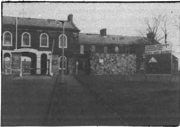
North-west District Armed Forces HQ, incorporating Regional Seat of Government 10, Fulwood Barracks, Preston.
