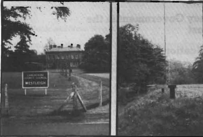
Westleigh, showing aerial and ventilation pipe emerging from the bunker at the back.
